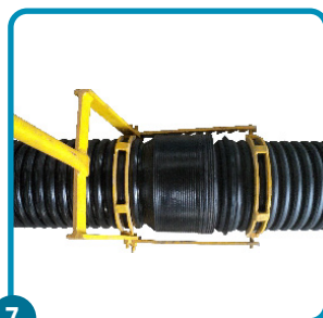
7 Bring pipe closer with joining device as shown in the picture
